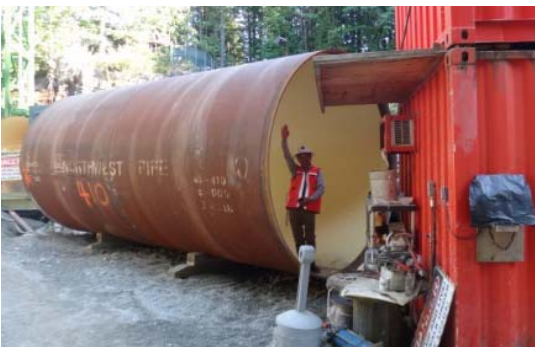
Michael Wu demonstrates the diameter of the water tunnel.
