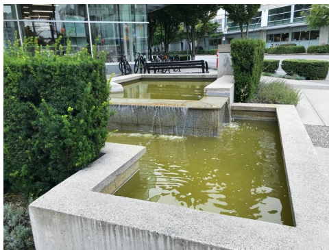
Figure 3— Decorative Water Feature (Did not pass inspection)
